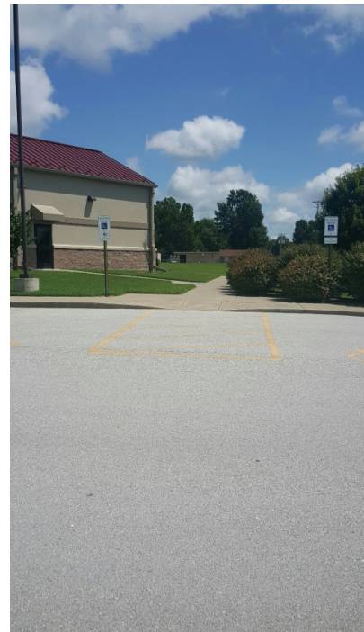
Image 18: Accessible Parking Space
