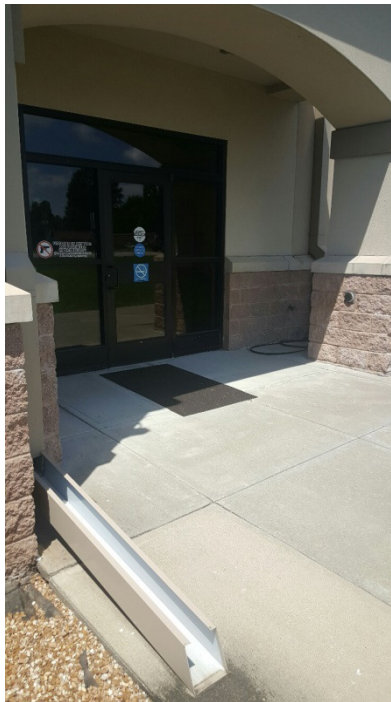
Image 17: Entry to Fire Station 1
