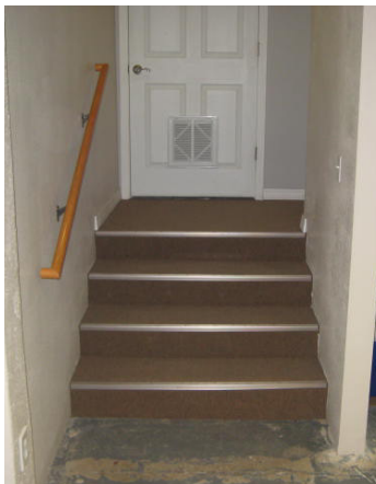
Image 7: Stairs within Primary Route
