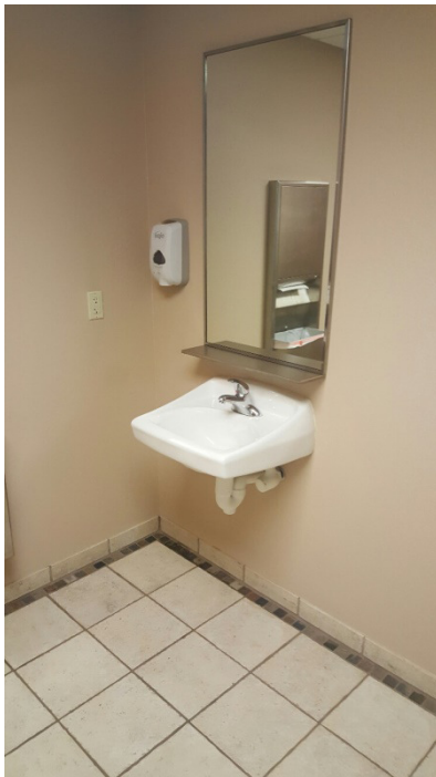
Image 16: Men's Toilet Room
