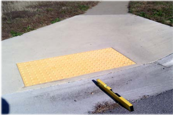
Ramp with truncated dome surface
