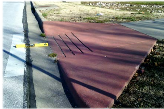
Ramp constructed in 2008
