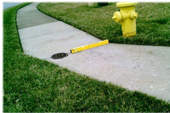
Sidewalk constructed in 2003
