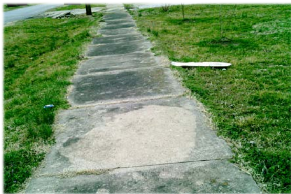
Sidewalk construction date unknown
