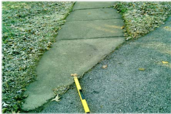
Ramp constructed in 1990
